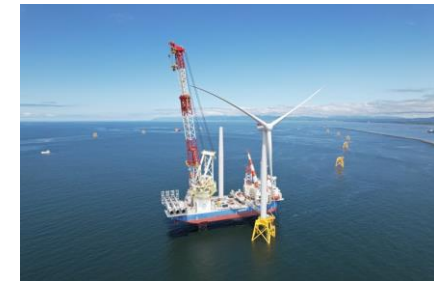
<Turbine Generator Installation>
